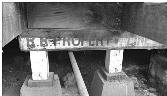
SP timber in foundation of Victorian house. (Fred Marsh photo)
